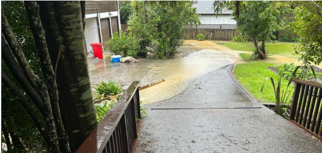
A pipe from under the road discharged stormwater into 37 Jocelyn Crescent ...
