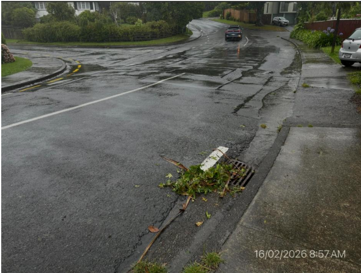
Figure 29 No flooding at Sunbrae Drive and Deller Grove intersection
