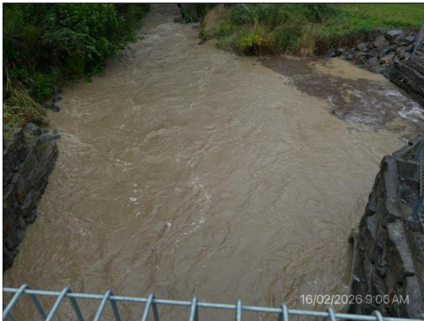
Looking upstream from the footpath above the intake
