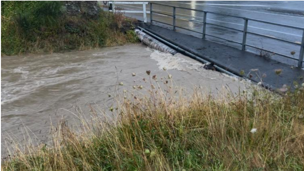
Field Street road culvert (upstream side) at 7:27am
