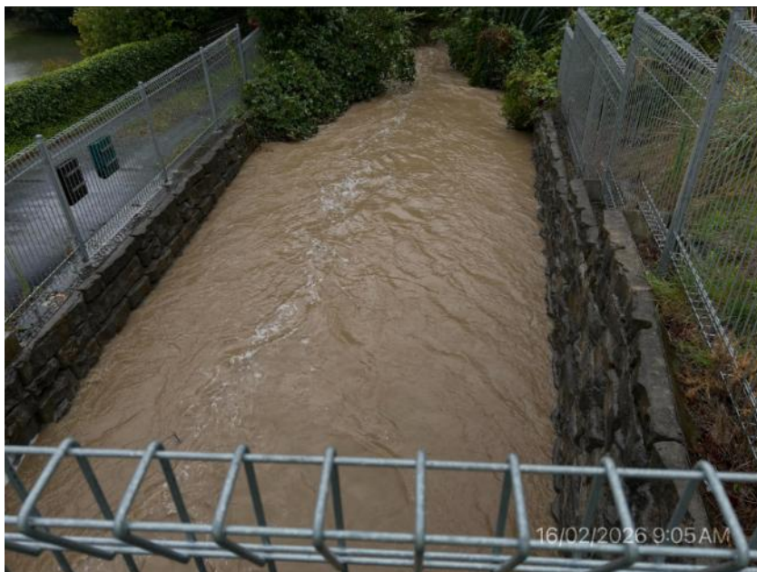
Looking downstream from the footpath above the new culvert outlet
