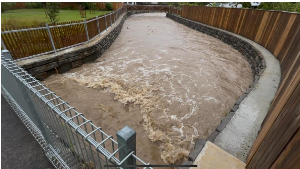
Figure 27 Sunbrae Drive new culvert, 8:51 am
