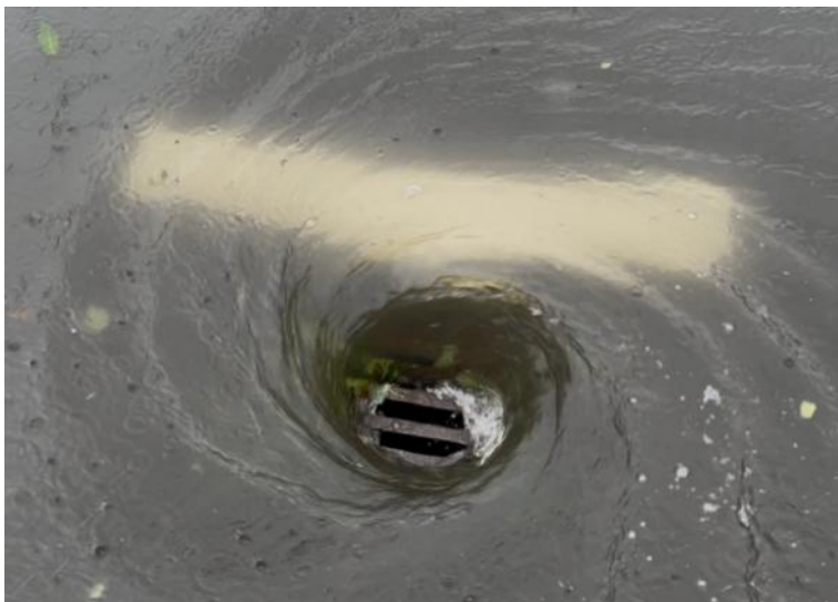
Figure 21 Ponding in Gard Street due to blocked road sumps
