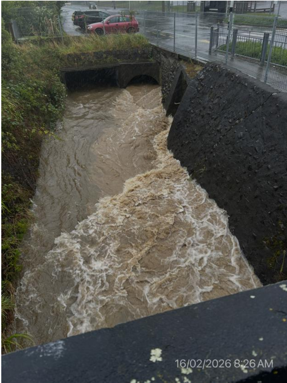
This photo (left) at 8:26am shows Hulls Creek at the time (approximately) of the peak flow of the Pinehaven Stream and Whitemans Road Bypass pipes
