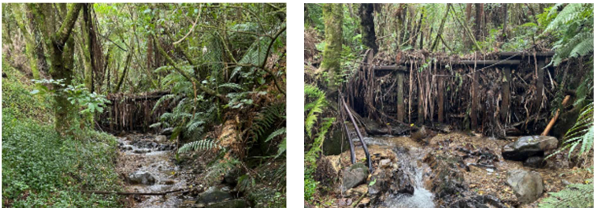
Figure 20 Upstream is a larger debris trap (both views looking upstream). Photos: FloodingUs NZ Ltd
