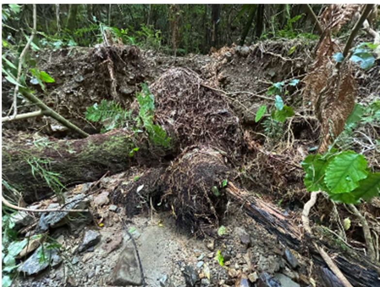
Figure 26 More examples of bank erosion upstream from the debris dam
