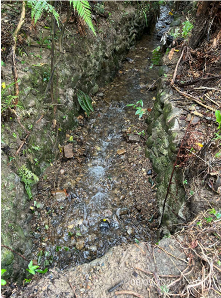
Figure 14 Photograph looking upstream at driveway culvert intake, 125 Pinehaven Road (Photo: 8 May 2026)
