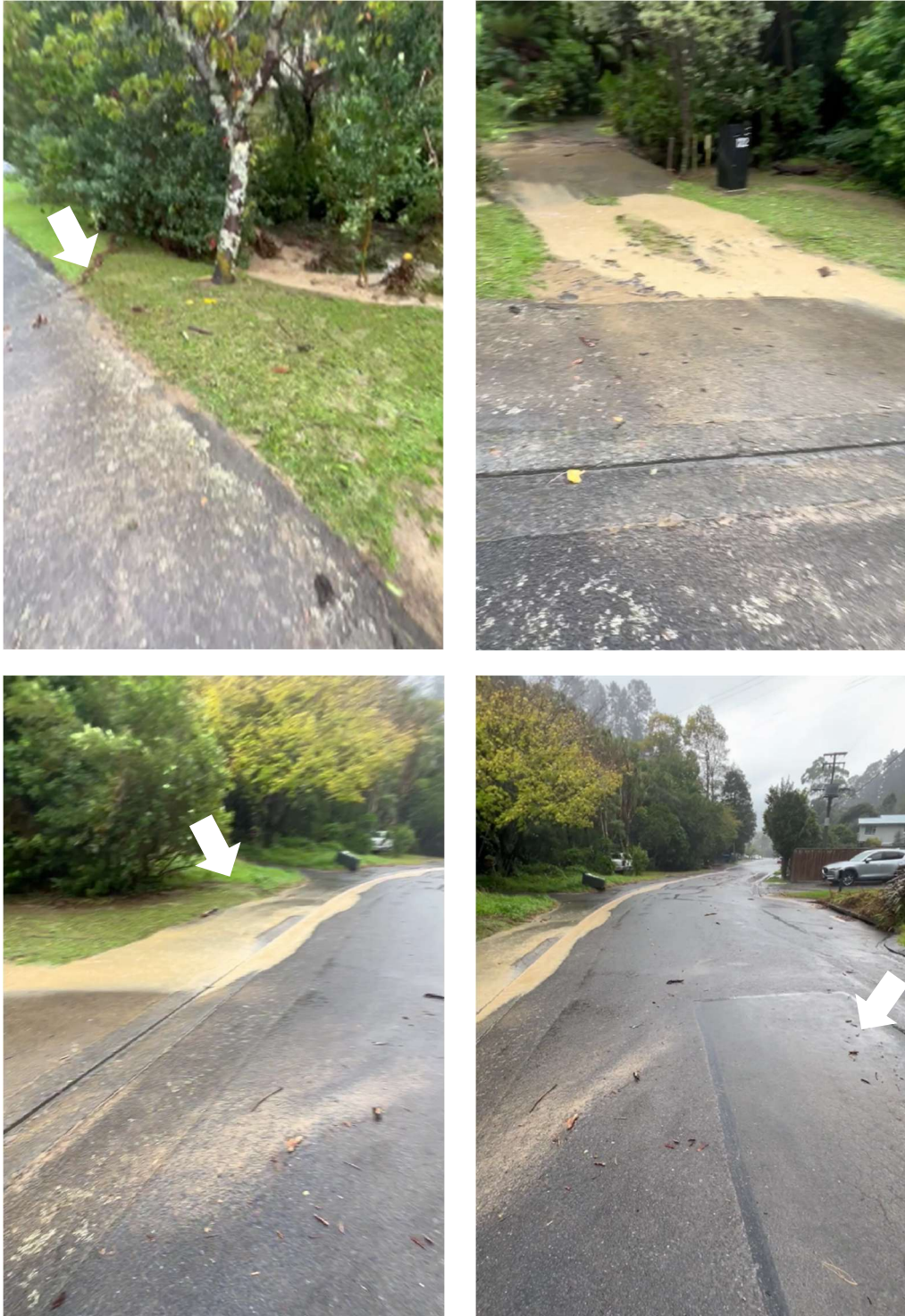
Figure 64 18-4-26 10:01am Debris from overtopped culvert 122 Pinehaven Rd
