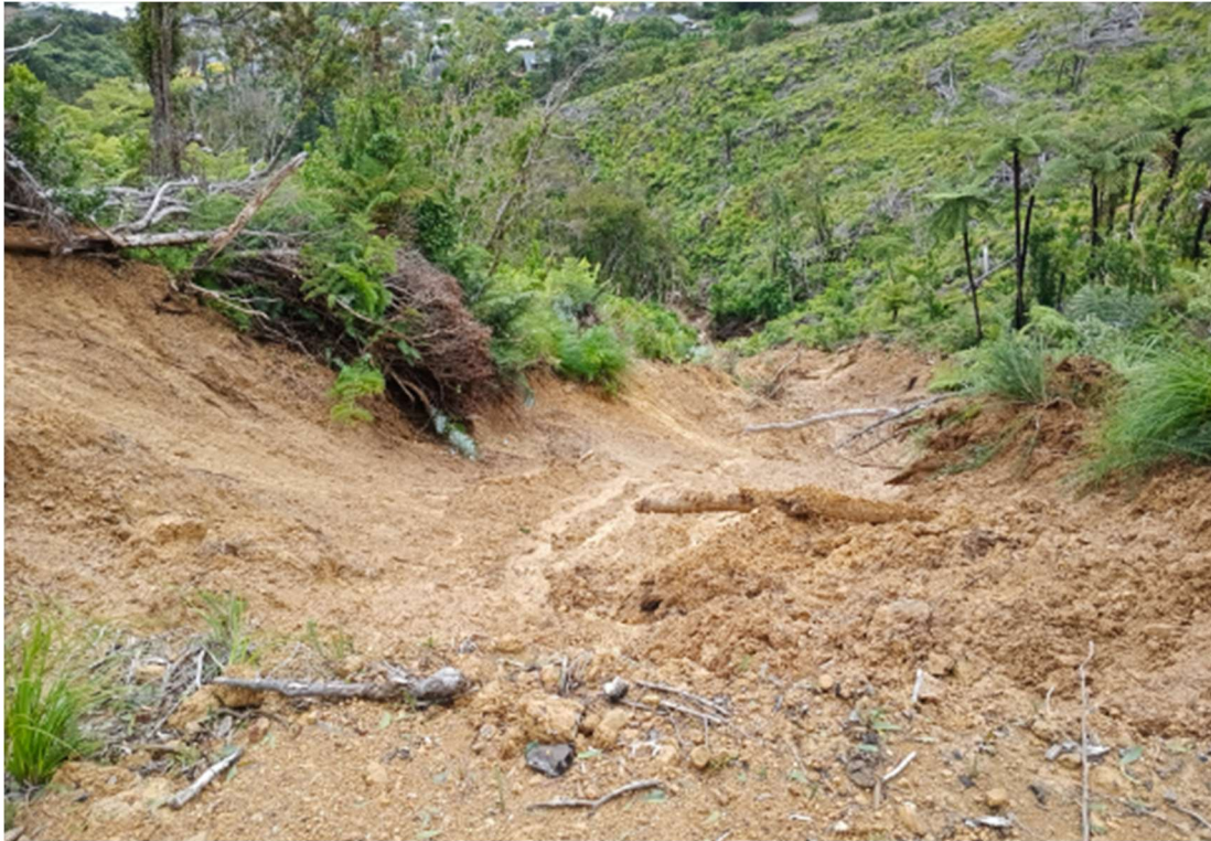
Figure 41 Landslide on steep GTC hills above housing in Silverstream (Photo: Dennis Clark)
