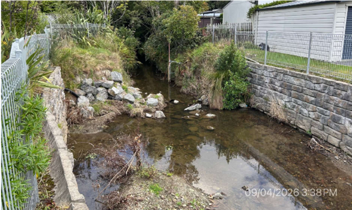
Figure 109 The rock pile on the True Left Bank was swept away in the 16 February 2026 event
