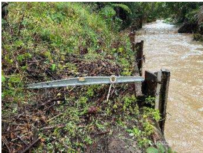
Figure 100 Measuring level of debris above retaining wall
