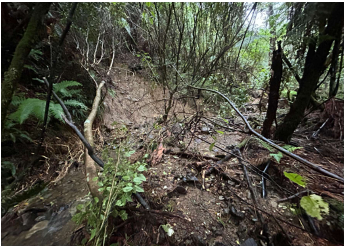
Figure 29 Much loose material in the stream bed, from scouring and erosion?
