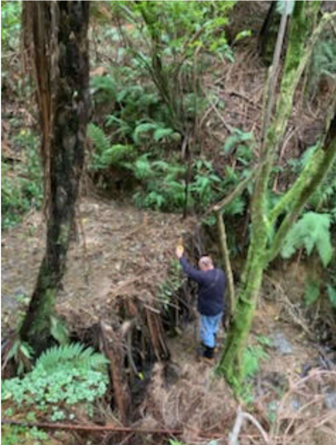
Figure 22 A debris dam 18 April 2026 raised the stream bed 1.6m. Photo: Flooding Us NZ Ltd
