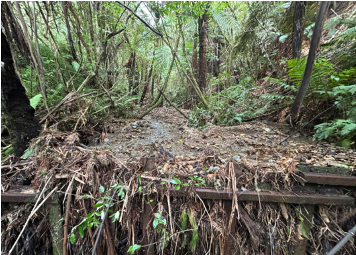
Figure 23 The debris dam - many tonnes of sediment, gravel, rocks and debris
