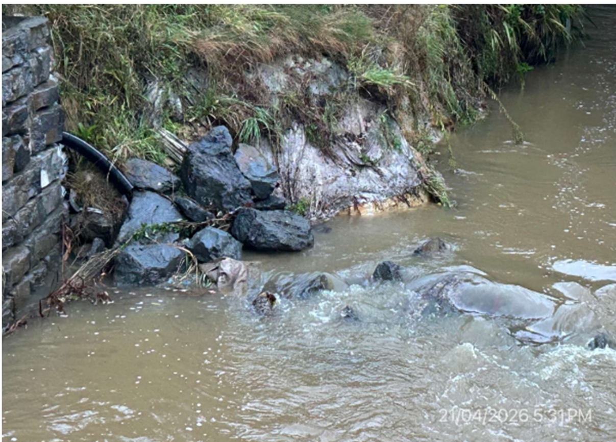
Figure 110 The rock pile on the True Right Bank was swept away in the 18 April 2026 event
